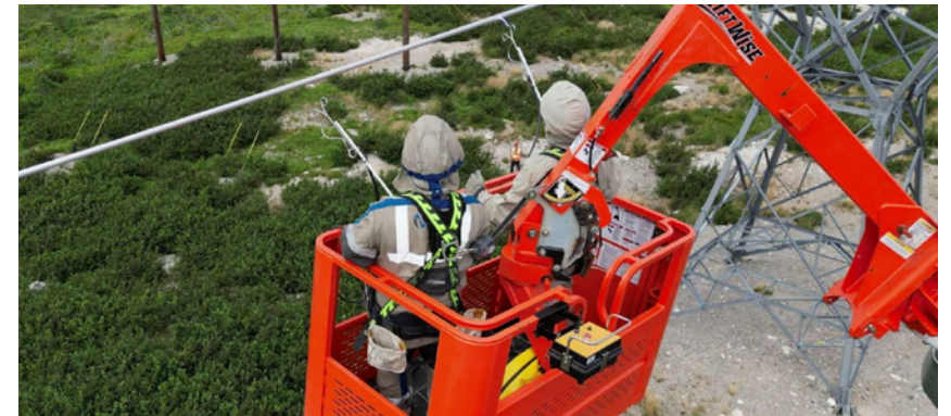
Two employees conducting live line work
