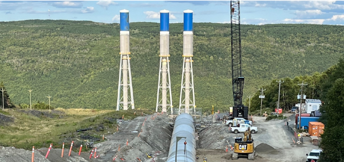
Penstock 1 replacement and refurbishment project at Bay d’Espoir
