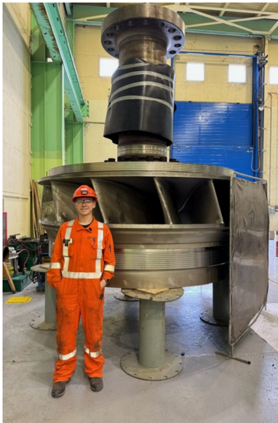
Alex Chaulk, Mechanical Graduate Engineer, standing next to disassembled Unit 1 turbine runner and shaft assembly in preparation for inspection.
