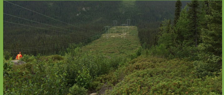
Members of the environment team perform an audit on the vegetation control program along the 230 kV transmission line near Churchill Falls.
