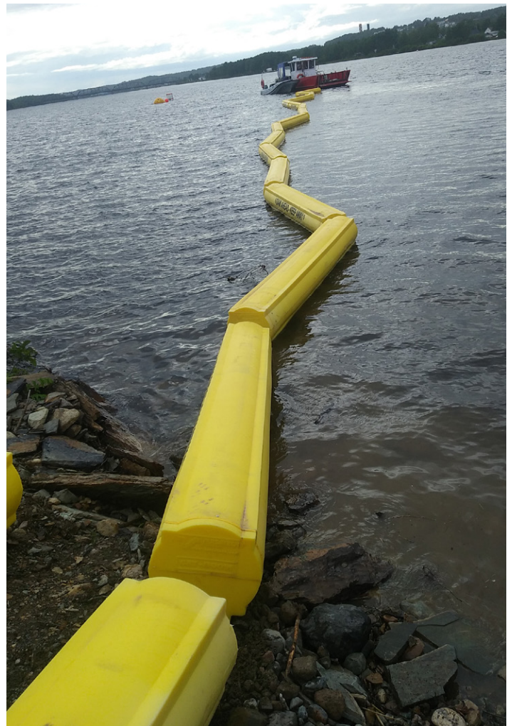
A safety boom in place at Bishop's Falls dam.
