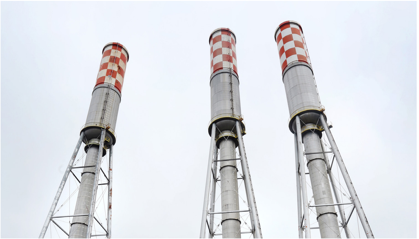
The surge tanks at Bay d'Espoir stand more than 370 feet above ground and were among the tallest in the world at the time of construction.
