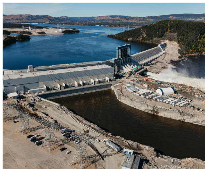
The powerhouse, spillway and north dam at the Muskrat Falls site.
