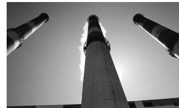
Photos above show construction of the Holyrood plant in the late 1960s. The smokestacks of units 1 and 2 are 91m tall and the stack on unit 3 is 110m tall.
