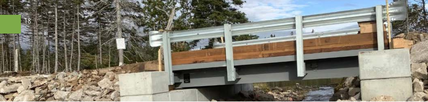
One of the newly installed bridges along LIL with erosion protection.
