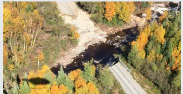
Top to Bottom: Long Pond Reservoir, Salmon River Spillway, road wash out resulting from Hurricane Igor.
