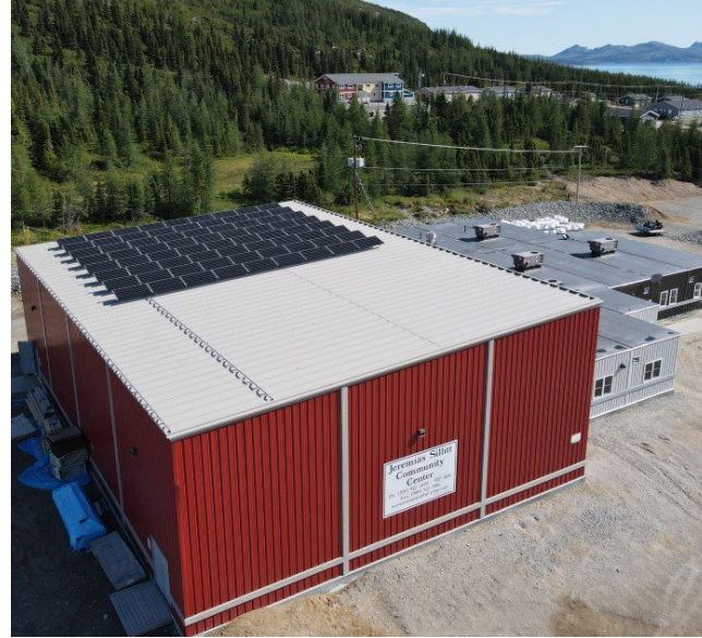
The Nunatsiavut Government completed four solar installations in Northern Labrador including the 24 kW system at the Nain JS Community Centre, pictured here.
