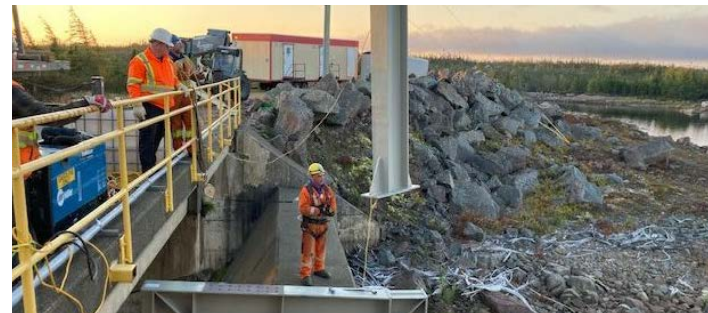
Our multi-year refurbishment project is underway at the Ebbegunbaeg Control Structure.
