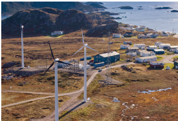
Wind Turbines at Ramea.
