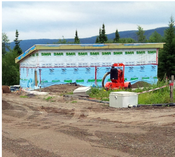
UV Disinfection Building.
