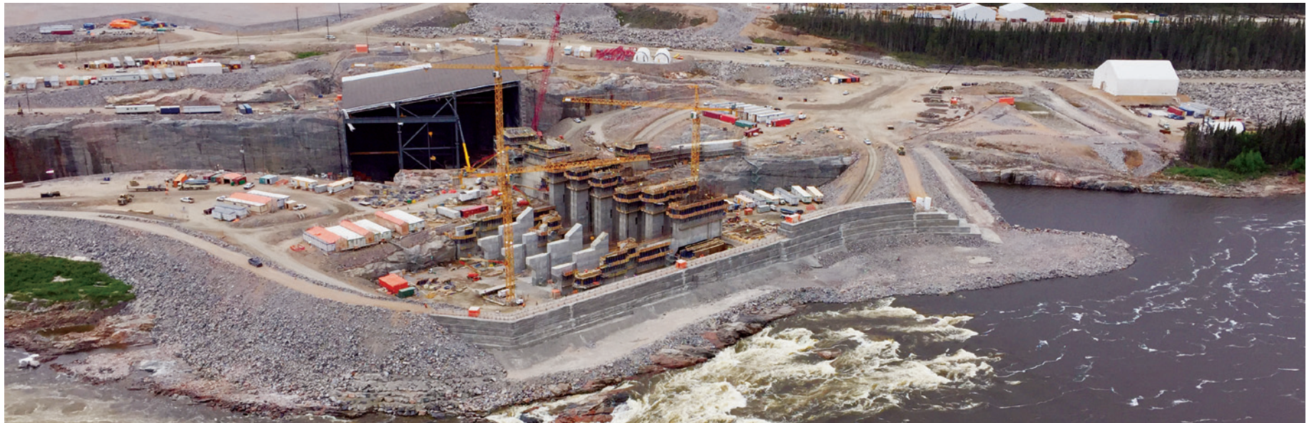
Spillway and power house excavation at the Muskrat Falls Site.
