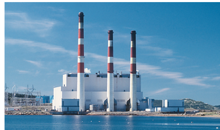
Holyrood Generating Station.
