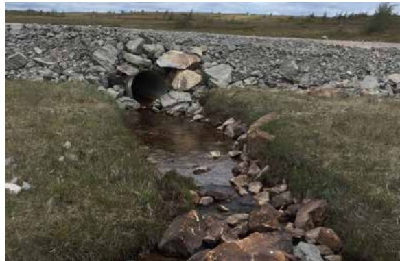
Culvert installation along the access for TL267
