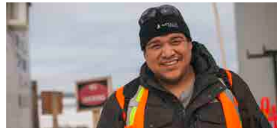
(TOP LEFT) Valard crew prepares final piece of transmission wire for stringing on the Labrador-Island Transmission Link
