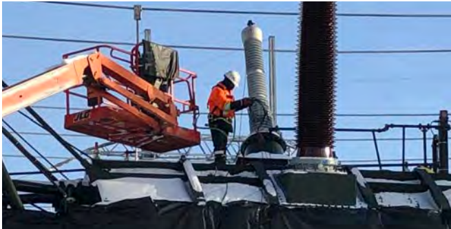
Installation of new transformer in the Churchill Falls Switchyard.
