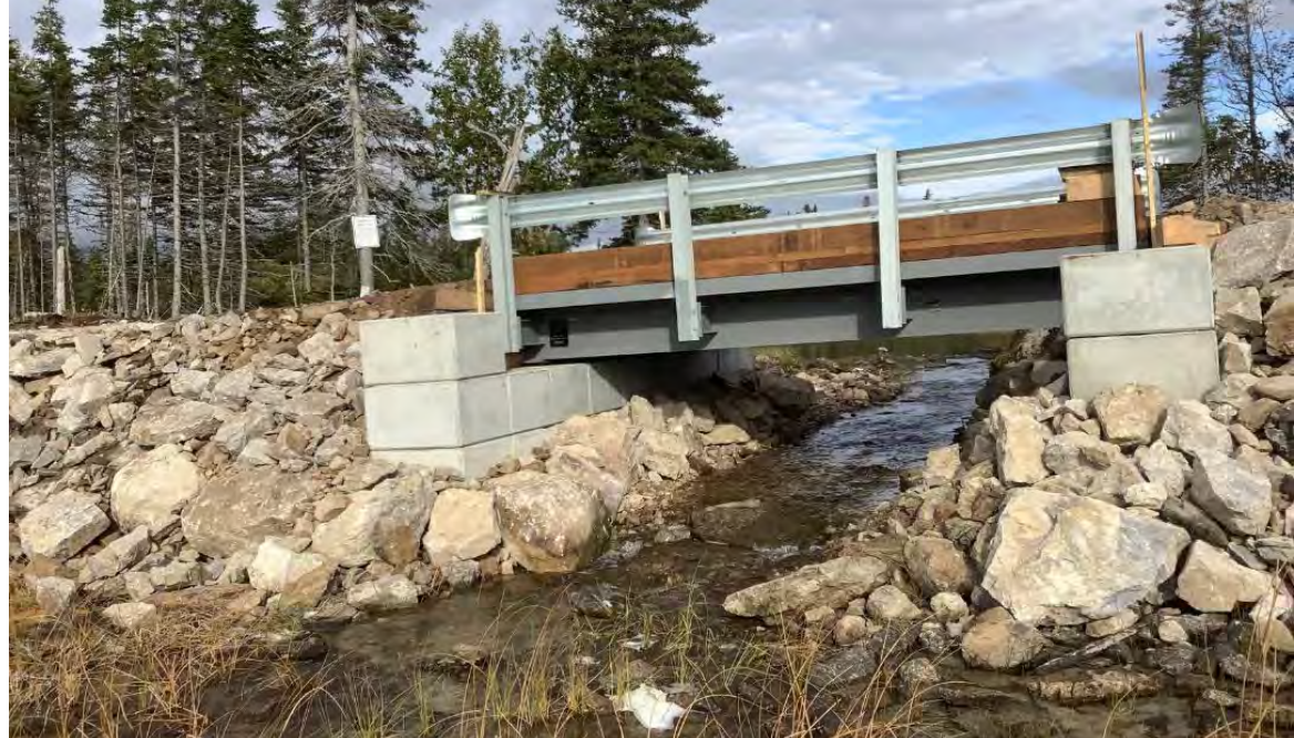
Newly installed bridge for LIL with erosion protection
