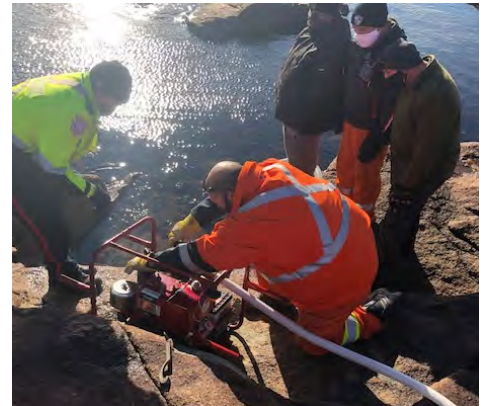
Matthew Brenton, Fire & Security Officer, ensures Black Tickle trainees get hands-on experience learning how to use their new emergency fire pump.
