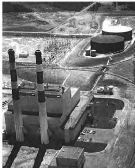
Photos above show construction of the Holyrood plant in the late 1960s. The smoke stacks of units 1 and 2 are 91m tall and the stack on unit 3 is 110m tall.
