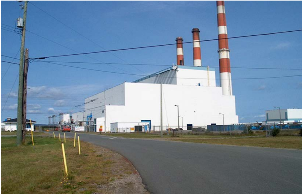
Figure 1: Holyrood Thermal Generating Station
