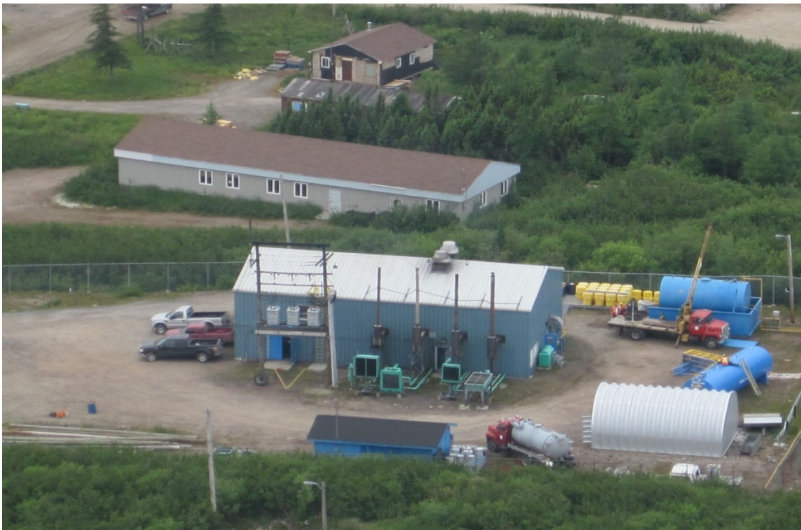
Figure 1: Cartwright Diesel Generating Station
